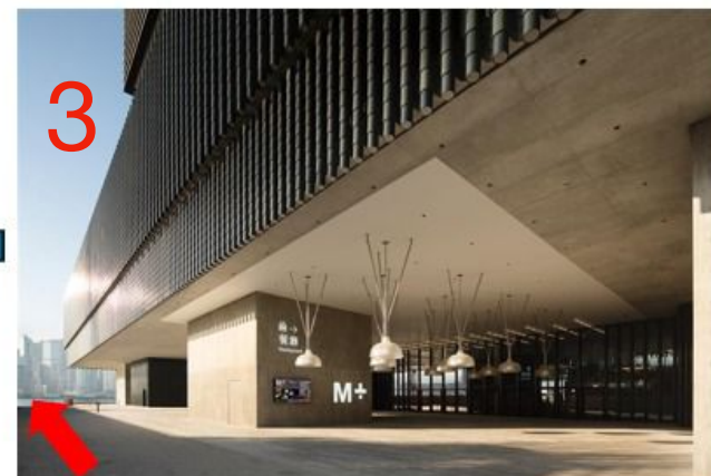
Go down the stairs located on the left side
